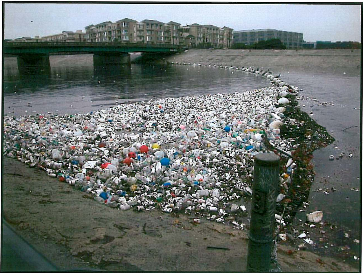
Trash net across typical Southern California Channel
