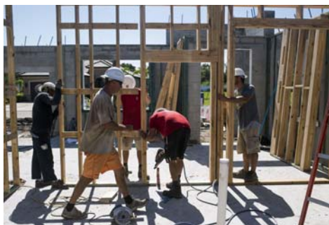
Workers installing wall frames at a home under construction in Ellenton, Fla., in July. PHOTO: TY WRIGHT/BLOOMBERG NEWS
