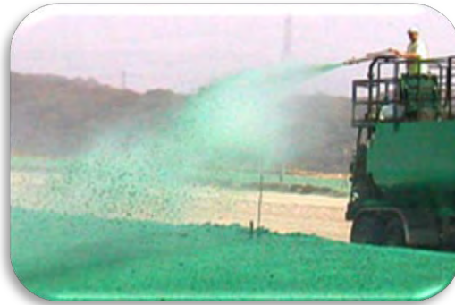
Figure 18 – Hydraulic Mulch Application. Source: California Department of Transportation < http://www.dot.ca.gov >
