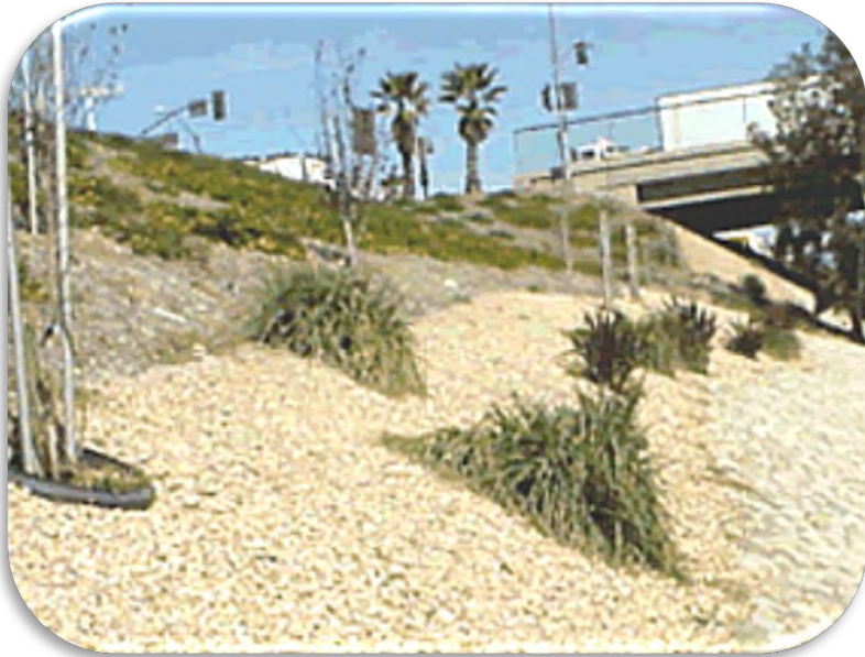
Figure 14 - Gravel Mulch Application. Source: California Department of Transportation < http://www.dot.ca.gov >
