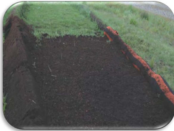
Figure 22 - Compost Blanket Application. Source: CASQA Factsheets, 2011.
