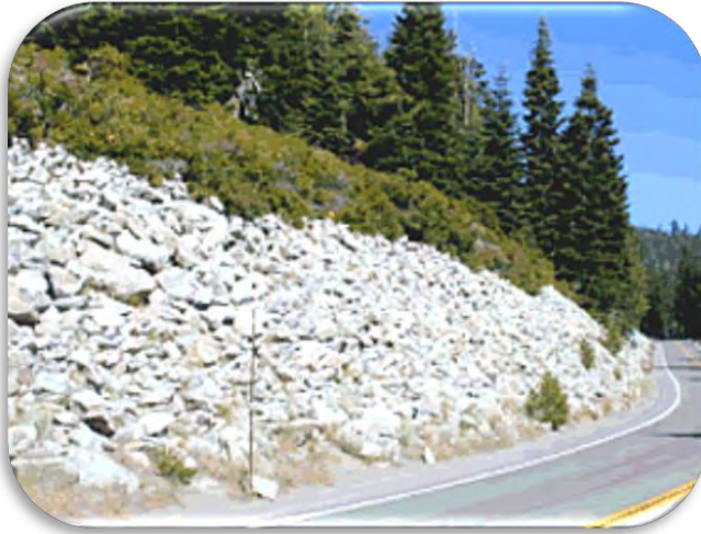
Figure 15 - Rock Slope Protection Application. Source: California Department of Transportation < http://www.dot.ca.gov >
