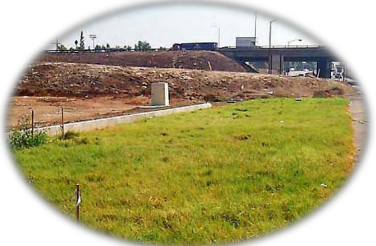
Figure 12 – Vegetated Filter Strip Application. Source: California Department of Transportation < http://www.dot.ca.gov >
