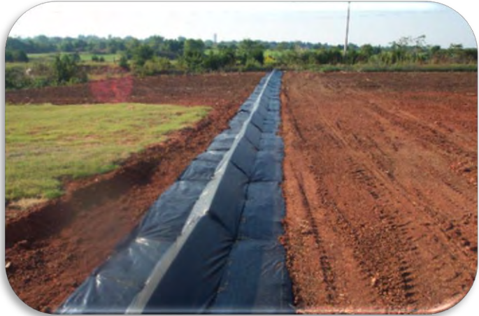
Figure 17 - Silt Dike Application. Source: http://www.tri-siltdike.com
