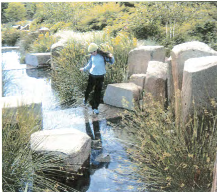
The Artful Rainwater Design system at the Oregon Convention Center Rain Garden in Portland controls stormwater runoff and allows visitors to interact with the water.
